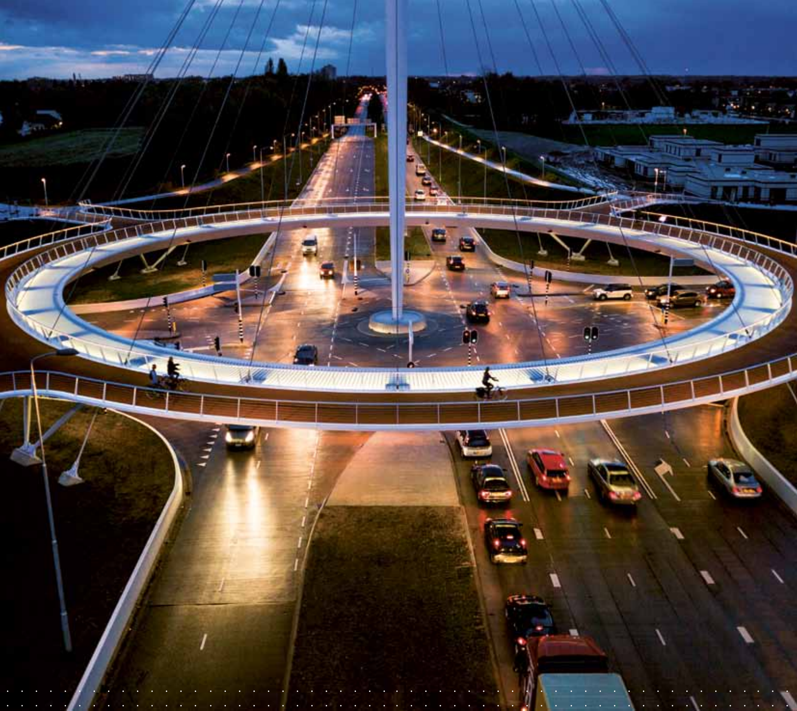
cds bicycle path coating on a tubular steel bridge, Eindhoven, NL
